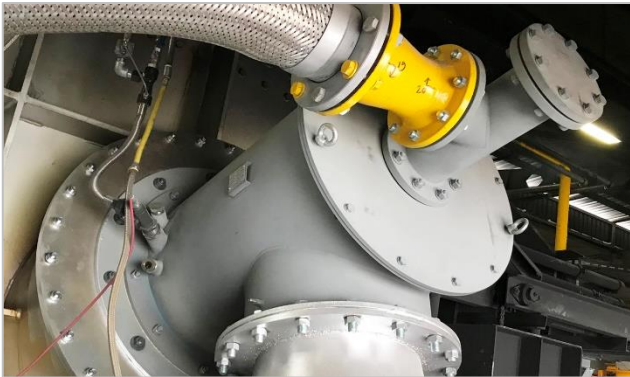
Copper Melting Furnaces
