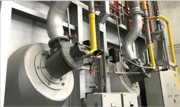
Aluminium Holding Furnaces
